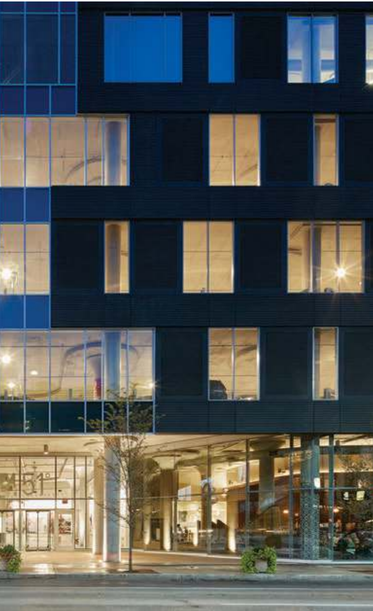
Three levels of above-ground parking at Cincinnati's 84.51° Centre were designed to become office space at a future date.
